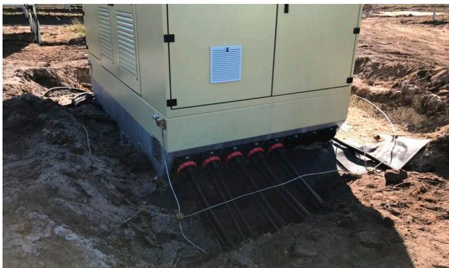
Depending of the performance of the different stations and the required number of cables several flanges were required. Due to the compact design of the flanges up to 7 can be installed in a row at the station floor. The installation of the supplied system cover HSI D3/58 as well as the sealing of the cable is done on site.
