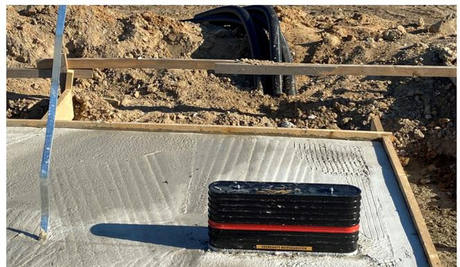
The multi-line building entry can be variably adapted to the finished floor level. The five flexible duct systems are laid up to the plot boundary. This means that trouble-free future retrofitting is also possible.
