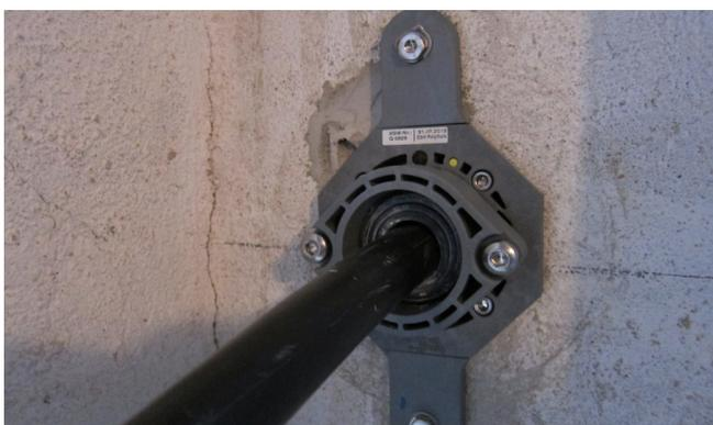
Final installation and resin-filled building entry with mechanical fixation and sealing element for electricity. Suitable for water or electricity media lines up to DA 50. Same sealing element design as for Hauff multi-line building entry.
