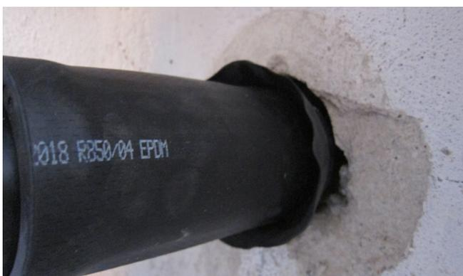
Following creation of an empty conduit route (DA 63) using a soil displacement rocket, the building entry is pushed into the core drill hole via the driving pipe.
