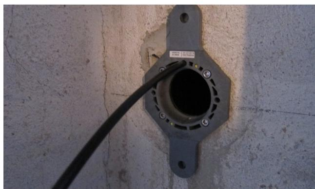
Fully inserted single building entry for trenchless construction with attachment tabs (mechanical fixing to poor-condition brickwork) prior to resin filling.
