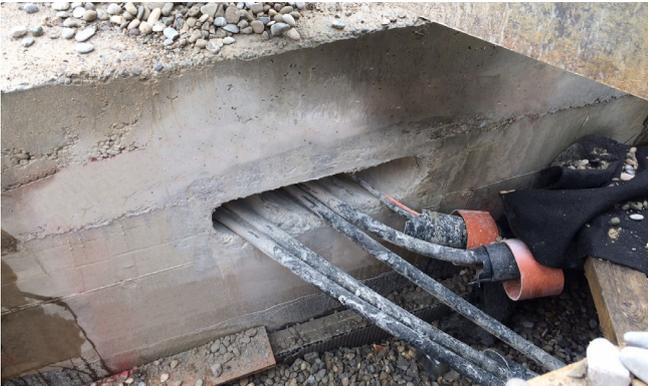
The existing main supply lines could not be rerouted during construction of an accessible service duct. A recess around the cables was left open during the construction work.
