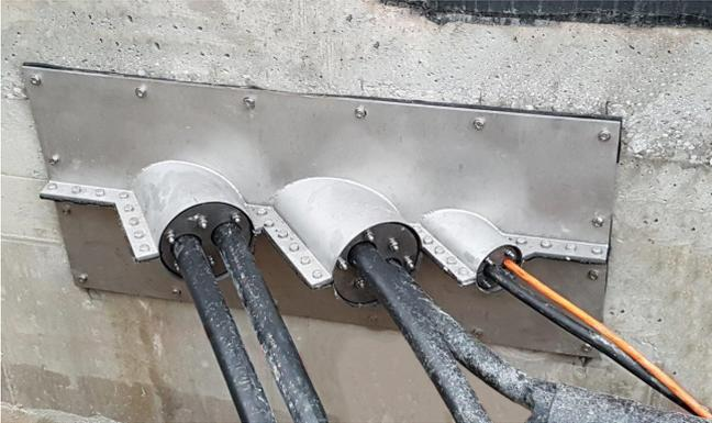
Solution: Overmeasure of a protrusion flange in split-design with different pipe socket outlets in relation to the exit angle of the cable.
