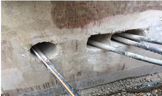
Special feature: Cables enter in and out of the service duct at varying angles. The position of the cables can not be altered.
