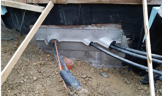
Image: Cable outlet on the service duct
