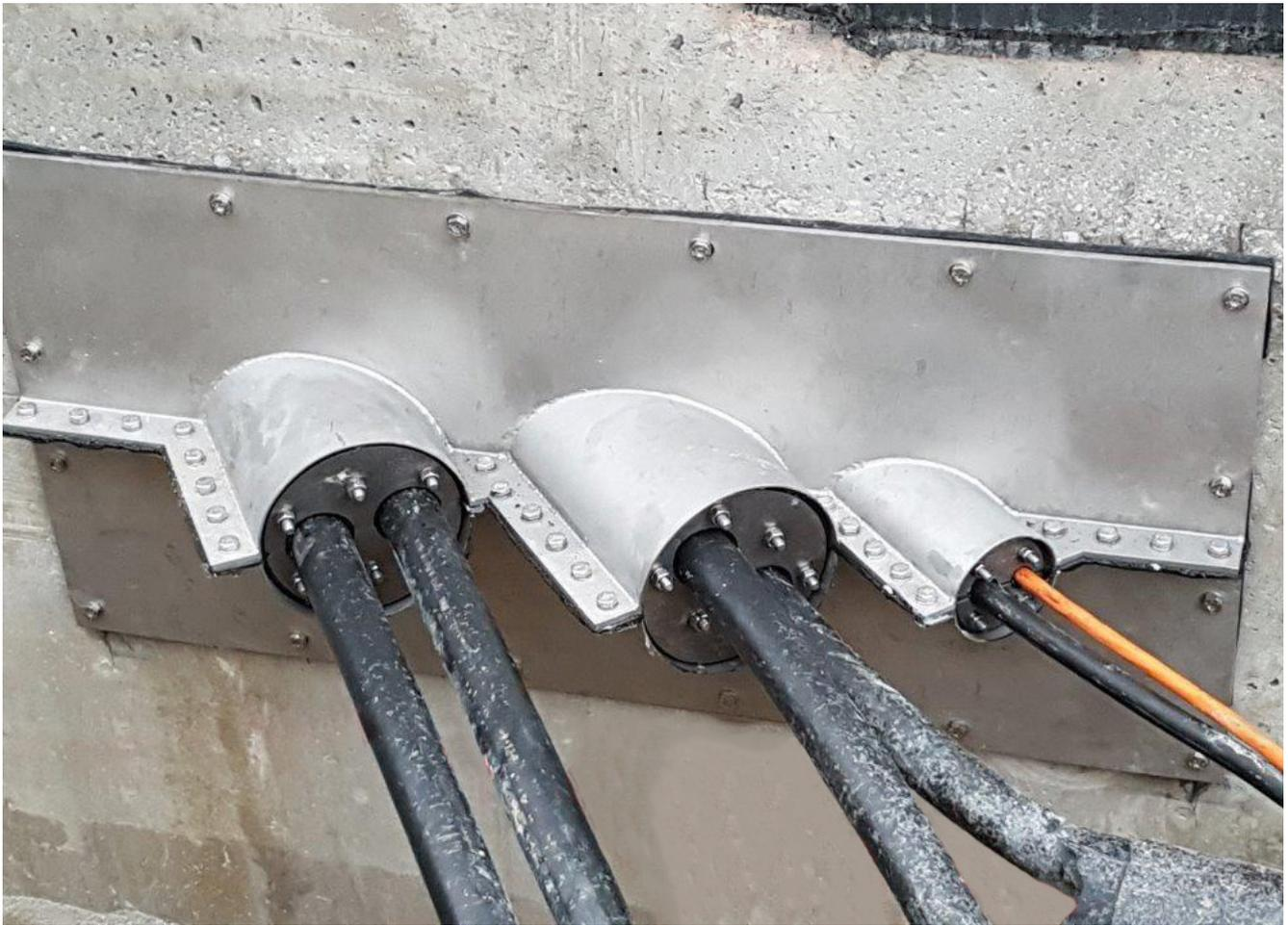
CABLE ENTRY WITH STAINLESS STEEL FLANGE HRD2X150-1X80
