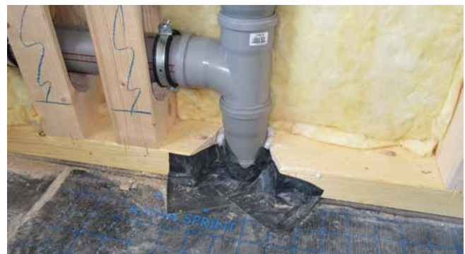
difficulty: integration of vapour barrier foil
