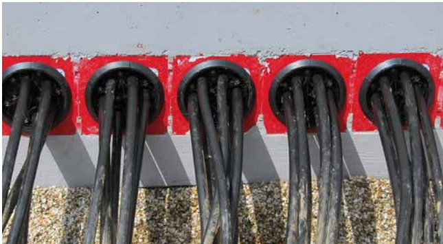
low-voltage cables sealed with HSI150 DG 6x10-36
