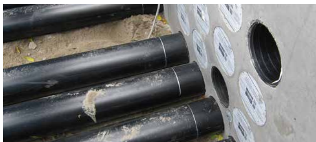
HSI150 GSM Varia applied as a block
