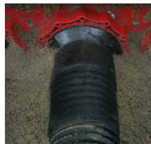
connection of corrugated pipes with cold shrink sleeves HSI150 D1x110 KS WR
