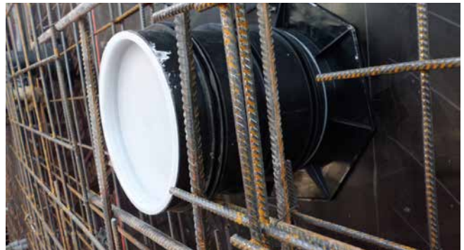
UFR in formwork
