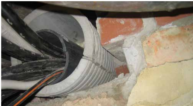
FZRG150/350 – refurbishment in masonry
