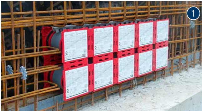
double wall insert HSI150 K2 before concreting
