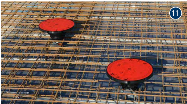
AT110 installed in the reinforcement
