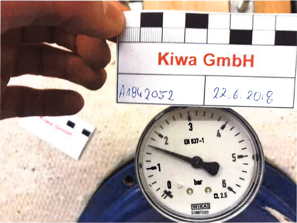
Figure A4. Water tightness test with \geq 1,5 bar water filled test cylinder (manometer after 24 hours on 22.06.2018).
