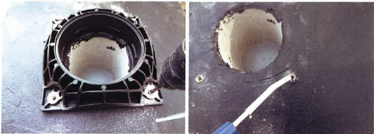
Figure 3. Drilling (left) und cleaning (right) of the dowel holes.
