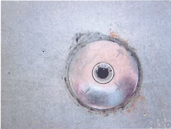
Illustration 17: Grounding penetration passage HEA-IS-M12/100, trough under-side after 92 days
