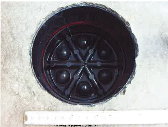
Illustration 4: HSI 150K/100 with HSI 150-D, concrete trough inner side
