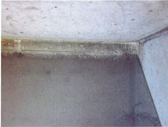
Illustration 11: Sheet steel base recess
