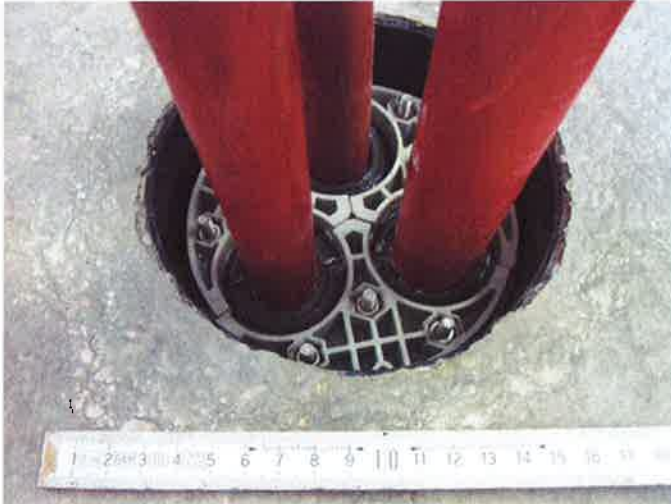
Illustration 3: HSI 150-DG, concrete trough inner side
