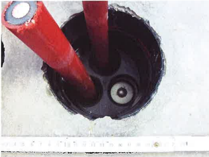
Illustration 5: HSI 150 D3/58 with seal plugs VS58/60, hot and cold shrink-on sleeve 150-K HSI 100, concrete trough inner side
