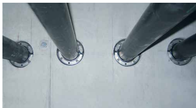
HSD125 1x75 b20 A2/EPDM55 raccordement de gaine
