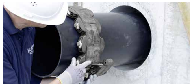
GKD400 – installation des segments
