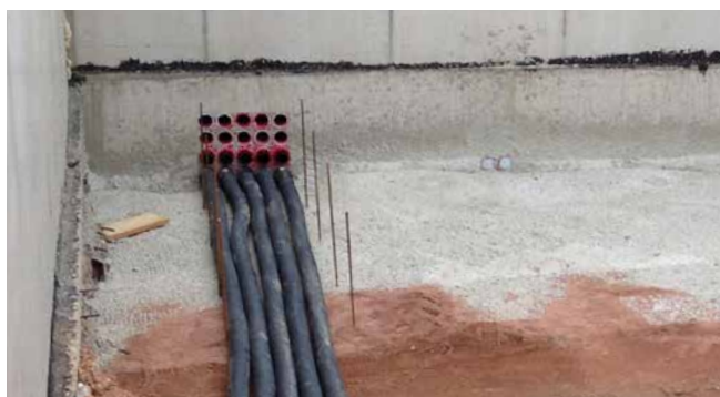
raccord de tube annelé HSI90 D1x75 KS WR
