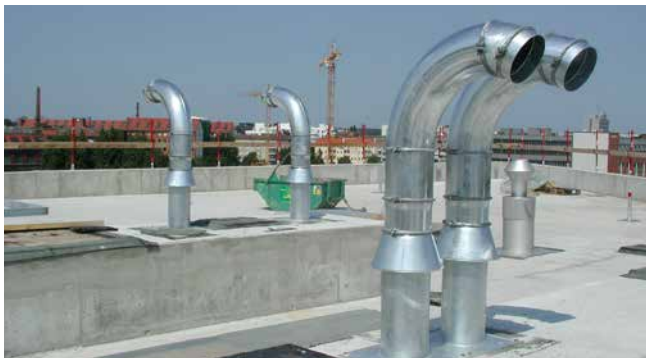
installed SHD200 before laying of cables
