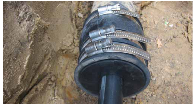
sealing set KES90 MA WE100 SG 1x18-65 SET for cable sealing at end of cable duct
