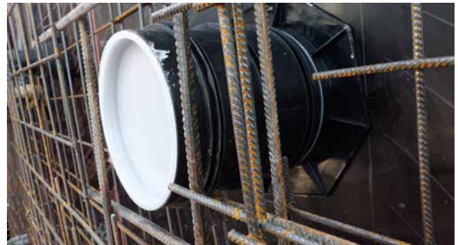
UFR in formwork
