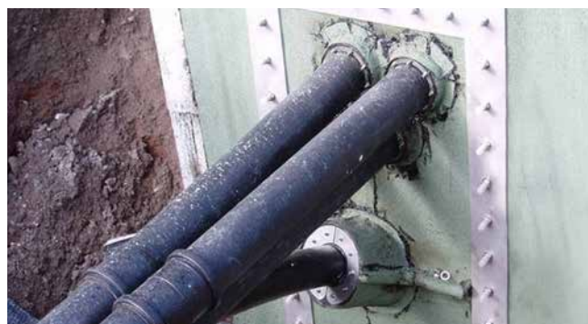
split fixed/loose flange according to DIN 18533
