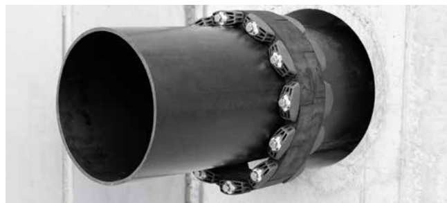
GKD400 – fully installed
