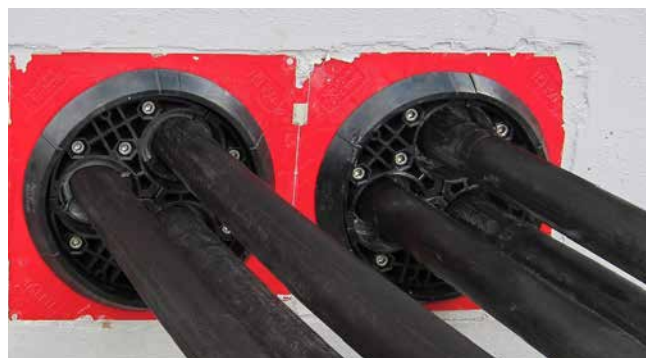
various installation stages for HSI150 DG 3x24-54
