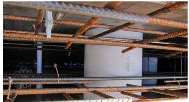
ZVR200/300 fixed in formwork
