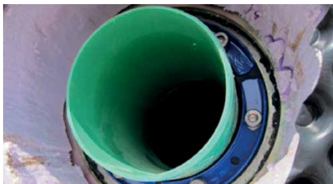
HSD150 C 1x110 b40 A2/EPDM55 in galvanised fixed/loose flange
