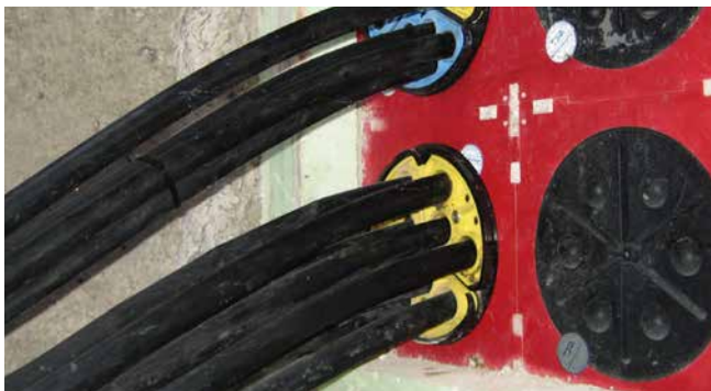
sealing of cables for street lighting with SEGMENTO
