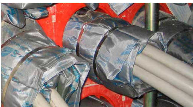
HSS – installation fire-stop pads in wall insert HSI150-K2, sealing with system cover or SEGMENTO
