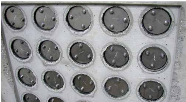
FZR100/240 – pipe section sealing
