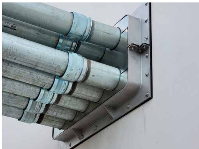
Stainless steel flange split for subsequent dowelling
