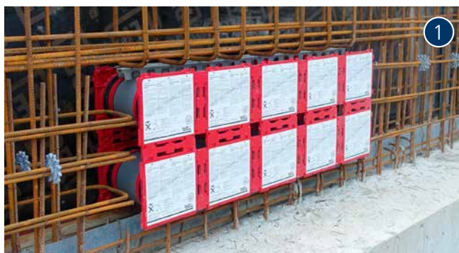
double wall insert HSI150 K2 before concreting
