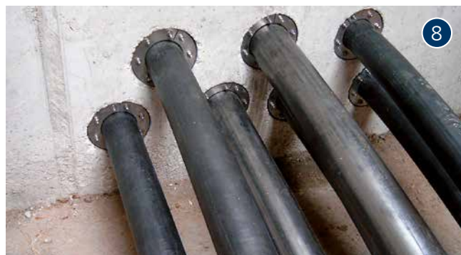
HRD press seals installed
