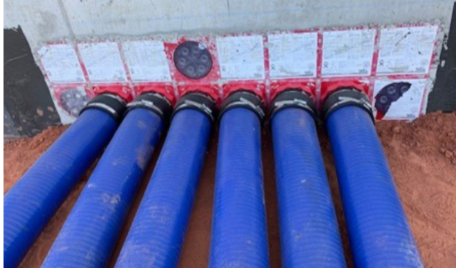
Connection of the Hateflex hose to the wall inserts is implemented via the KES MA150 D system cover.
