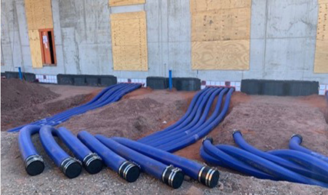
Thanks to its characteristics such as dimensional stability, kink resistance, suitability for building-over, weather and UV resistance, Hateflex spiral hose offers the ideal conditions for the safe and gentle laying of cables.
