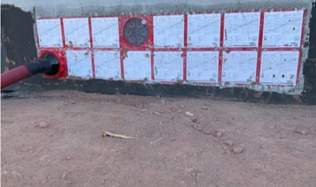
In the number of cable entries with HSI150 K2/x double wall inserts, a sufficient number of reserve openings has been taken into account.
