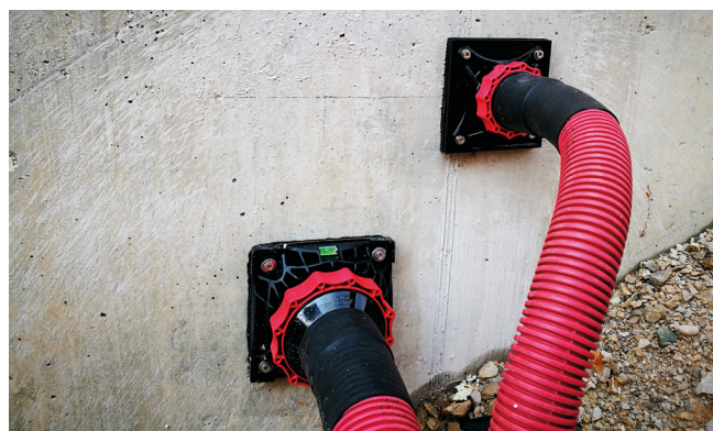
Vgrajene uvodnice HSI 150-DFK s sistemskimi pkrovi HSI 150-D110 KS, HSI 150-M168 WR in HSI 150-DG-3/24-54.
