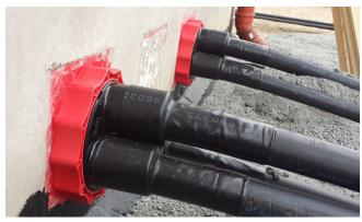
Underground cables sealed with shrink technology
