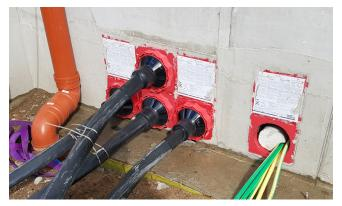
Underground cables sealed with shrink technology
