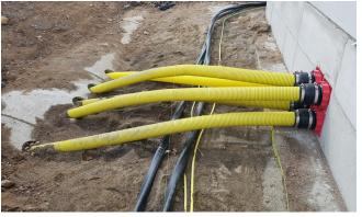
Duct connection with HSI 150 rubber sleeves
