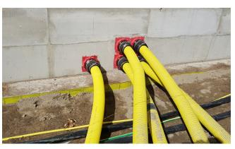
Duct connection with HSI 150 rubber sleeves
