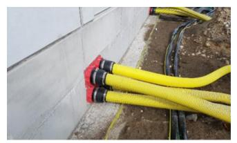
Duct connection with HSI 150 rubber sleeves
