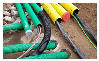
ADS to seal ducts inside core drills
