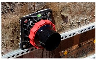
HSI system cover is then simply attached via the bayonet system to the DFK and tightened by the red clamping nut.
