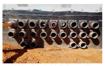
KME trialled three to begin with, the builder then approved the system and completed another layer of the membrane. New cole-holes were drilled then another twenty two HIS 150-DFK and system covers were installed after early success and ease of installation.
