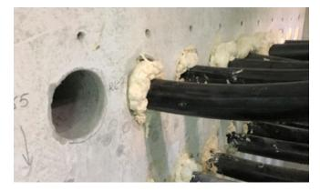
Within the basement of the residential tower, cables with different diameters were installed in core drilled holes.
