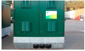
Due to the lightweight design using metal sheet floors instead of concrete, the transformer stations can be transported by large trucks from Germany to Southern Spain
