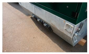
The glass fibre reinforced flanges for retrofit dowelling were already pre-installed by the manufacturer of the transformer housings and closed with a HSI 150-D blind cover. For installing the HSI flanges on the metal sheet floor metal screws were used (according to the material thickness of the floor. Screws were provided locally).
