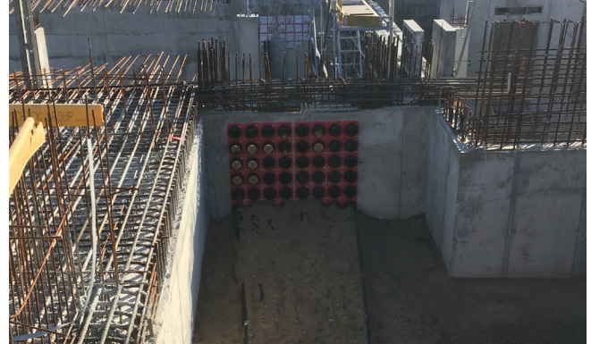
Smooth cable ducts with a diameter of 160 mm were attached to the cable entries in layers with HSI150 M168 system covers. The snapshot shows the first layer of cable ducts.
