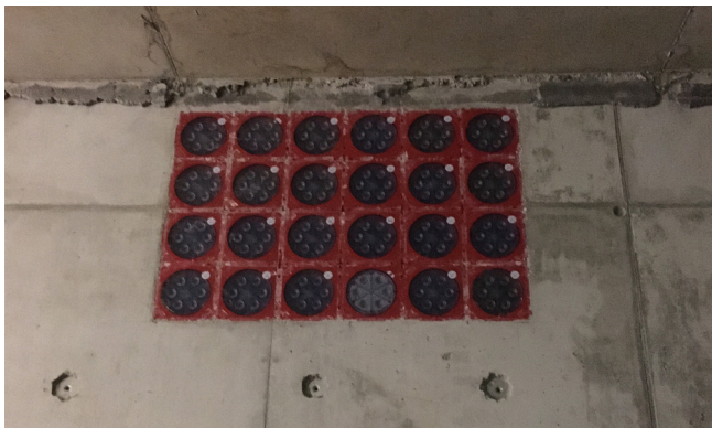
Vacant cable entries are already permanently blind sealed to a pressure of up to 2 bar. Thanks to the transparent HSI150 DT closing cover, any water ingress in the cable entry or cable duct can be seen at all times.
