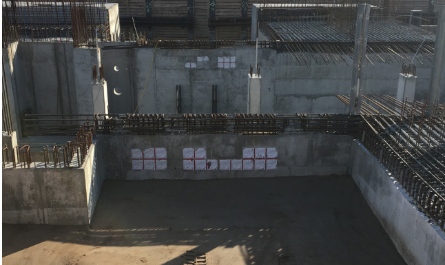
The HSI150 K2 cable entries from Hauff-Technik were used for connecting cable ducts and for subsequent sealing of the cables.
