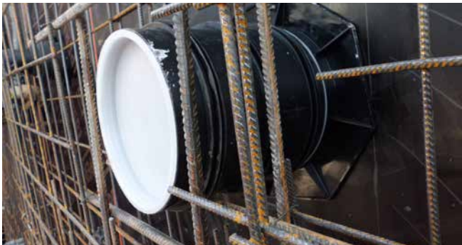
UFR in bekisting
