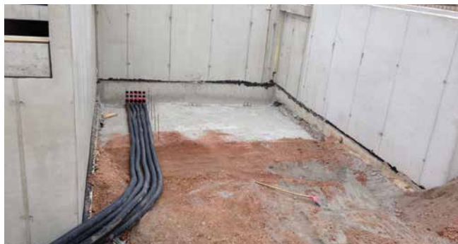
geribde mantelbuizen HSI90 D1x75 KS WR
