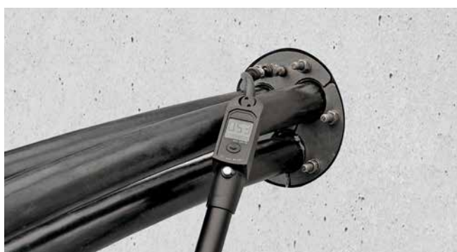
HRD150 PV G in kernboring
