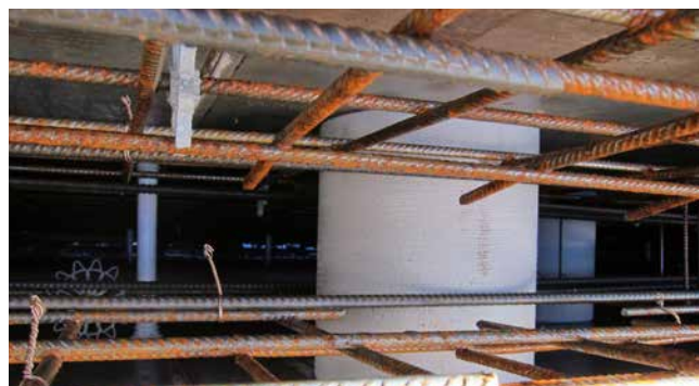
ZVR200/300 in de bekisting vastgezet
