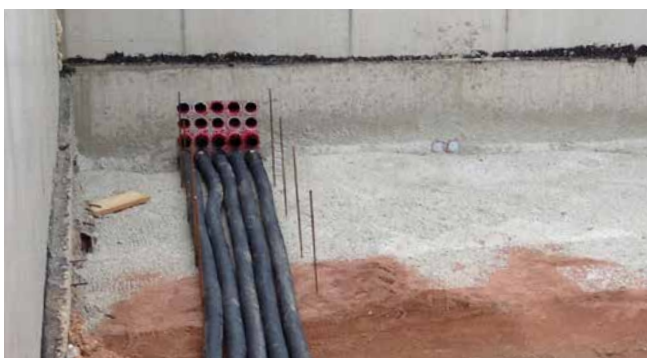
geribde mantelbuizen HSI90 D1x75 KS WR
