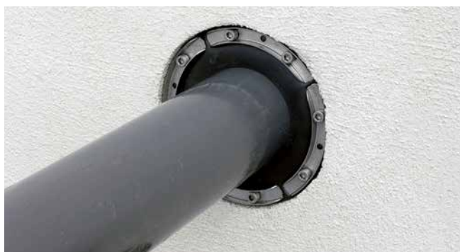
HSD200 1x159 b20 A2/EPDM55 "schachtafdichting"
