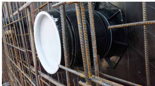
UFR in bekisting
