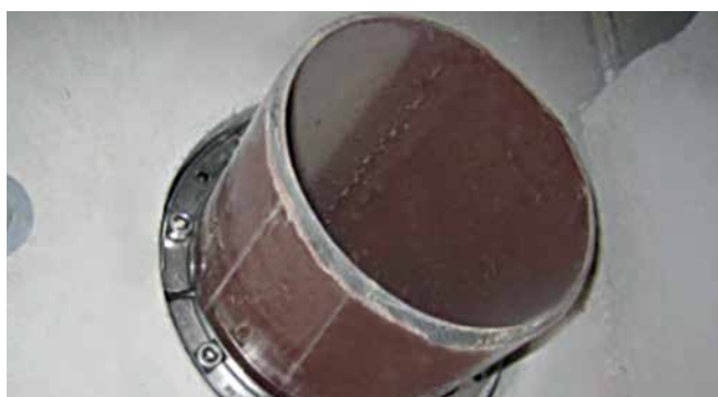
HSD200 1x160 b40 A2/EPDM55 – afwatering SML buis
