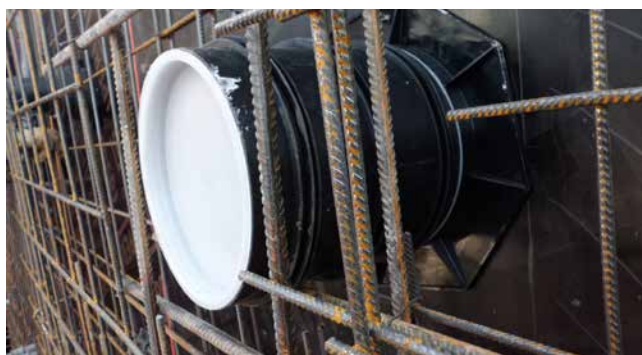
UFR in bekisting
