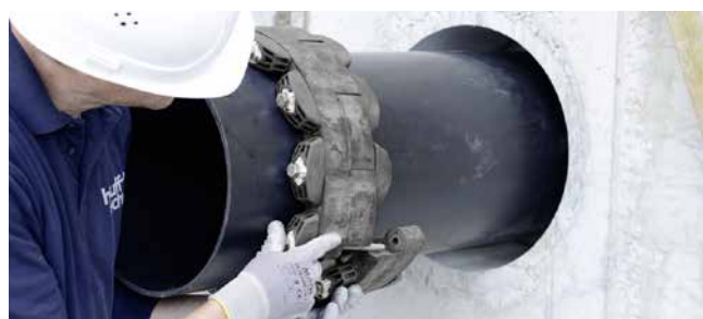
GKD400 – installation des segments
