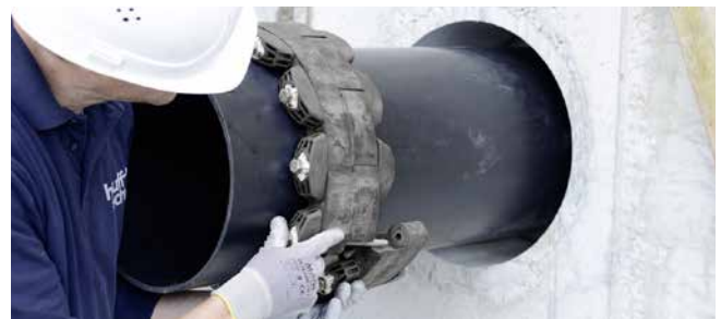
GKD400 – installation des segments
