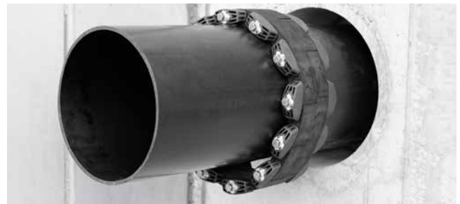
GKD400 – installation fini
