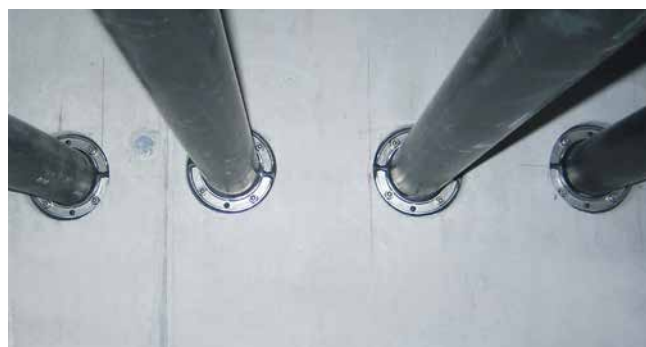
HSD125 1x75 b20 A2/EPDM55 raccordement de gaine
