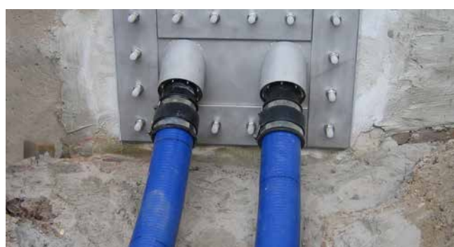
HSD b40 installé
