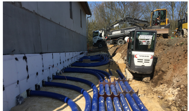
The HSI150 wall inserts set in the concrete are gas and watertight. They are located inside the concrete wall, behind the building insulation. The hose is connected to the wall inserts via the KES-M 150-D system cover.
