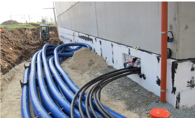
The rigid Hateflex14150 cable duct system is mechanically pressure resistant and provides for the relevant bend radius.
