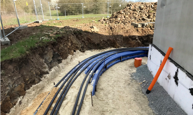
Precise fixation of the Hateflex spiral hoses with KES150-2x3 KA spacers for optimal soil compaction and subsequent laying of cables.
