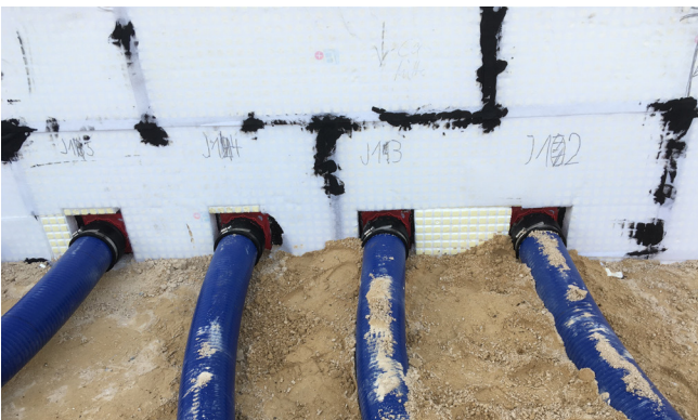
The Hateflex14150 spiral hose is connected to the concreted HSI150 cable entries gas and watertight using a rubber sleeve method.
