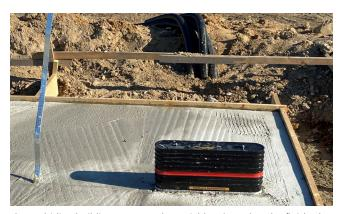
The multi-line building entry can be variably adapted to the finished floor level. The five flexible duct systems are laid up to the plot boundary. This means that trouble-free future retrofitting is also possible.
