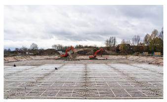
The horizontal collectors were laid beneath the construction field.
