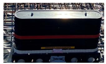
The basic insert of the MSH Basic FUBO R5 multi-line building entry is aligned to the profile board and prepared for concreting of the floor slab. At the Neustadt residential area development, the five-line floor entry is used for the following utilities: local heating feed and return, drinking water, electricity and telecommunications.
