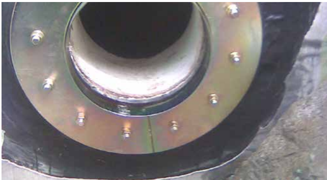
FLFA 1x400/X A3C drainage connection
