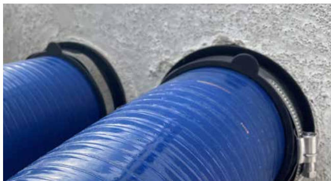
HSI150 KMA instalado
