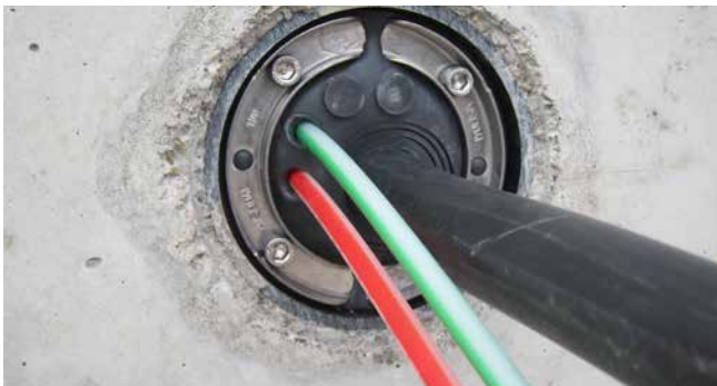
HSD100 EW instalado
