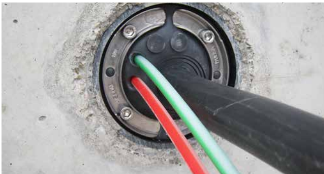
HSD100 EW instalado
