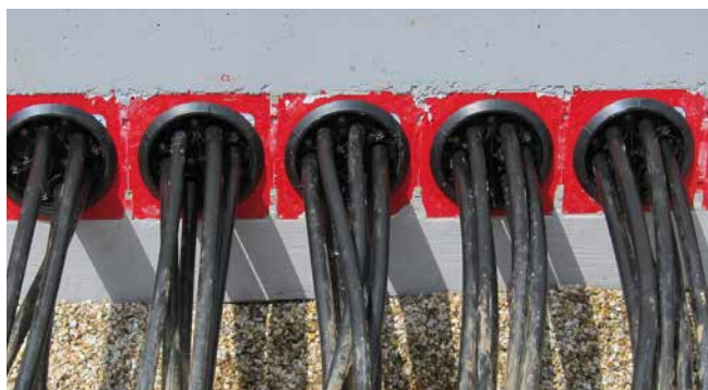
low-voltage cables sealed with HSI150 DG 6x10-36
