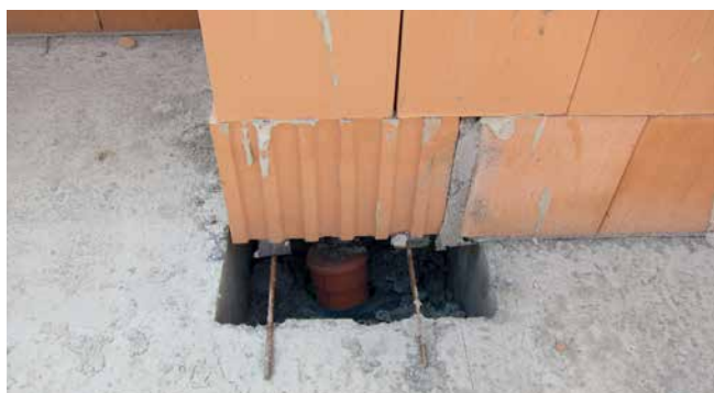
difficulty: retrofit gas-tight and vapour-proof sealing
