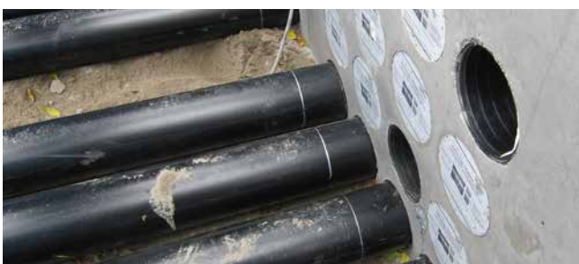
HSI150 GSM Varia applied as a block
