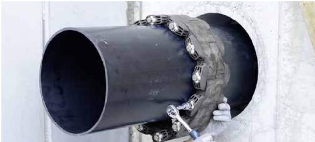
GKD400 – tightening of segments
