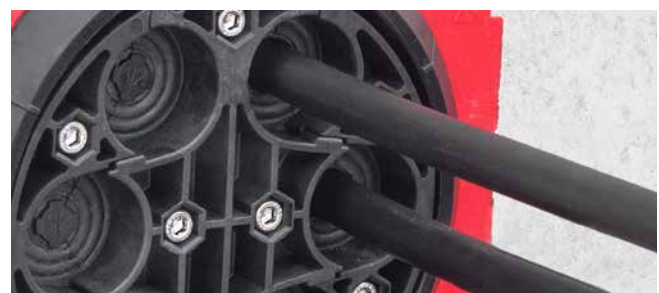
sealing with system cover HSI150 DG
