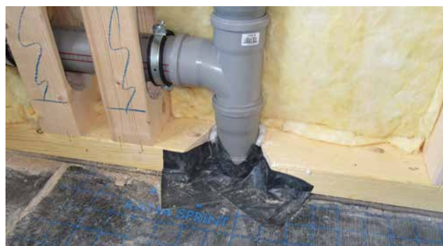
difficulty: integration of vapour barrier foil
