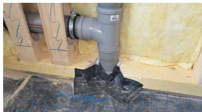
difficulty: integration of vapour barrier foil
