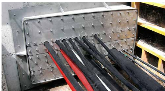
rectangular split flange for several cable penetrations
