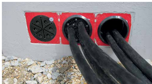
various installation stages for HSI150 DG 3x24-54
