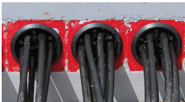
low-voltage cables sealed with HSI150 DG 6x10-36
