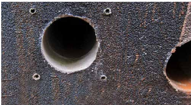
core drill and dowel holes
