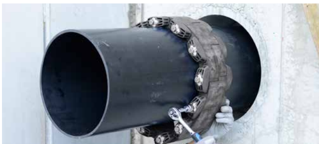
GKD400 – tightening of segments
