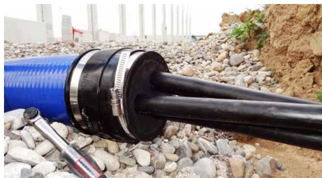
sealing in soil at the end of spiral hose Hateflex14150 with the sealing set KES150 MA WE 160 SG 3x22-58 SET
