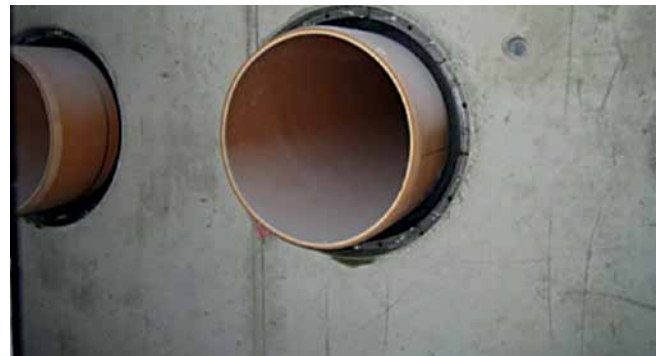
HSD500 G 1x429 b40 A2/EPDM55 – ventilation and air extraction
