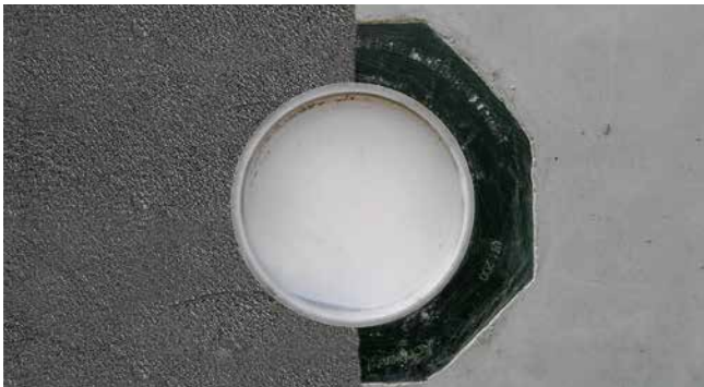
concreted UFR with PMBC
