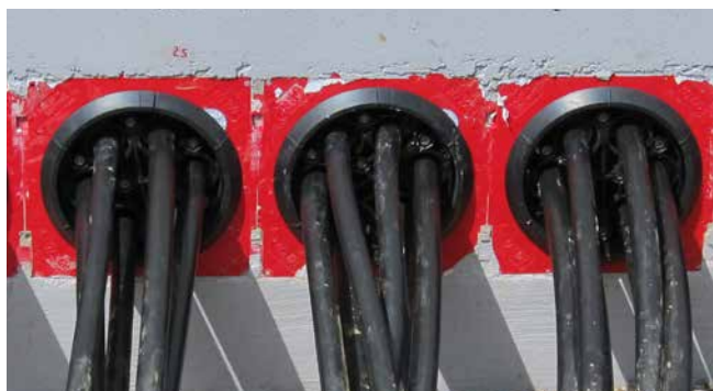
low-voltage cables sealed with HSI150 DG 6x10-36
