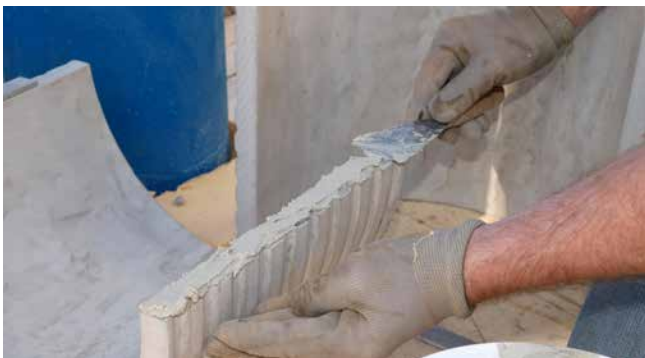
FZRG350/300 with levelling compound from installation set MSET FZRG
