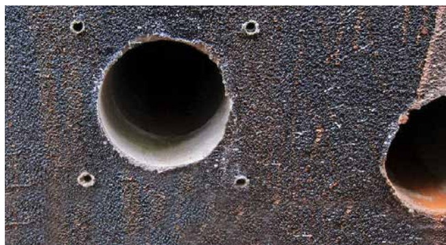
core drill and dowel holes
