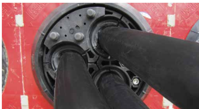
pressure plate cover HSI150 DG PA 3x24-54
