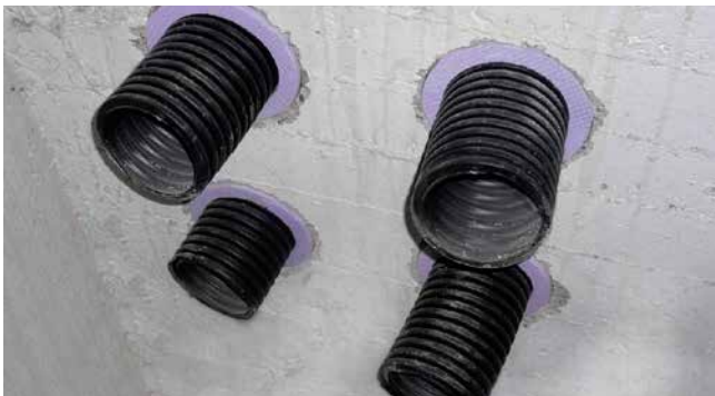
view of inside of building (insulation ring)
