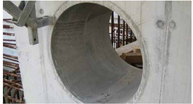
FZR400/300 – installation in water treatment plant
