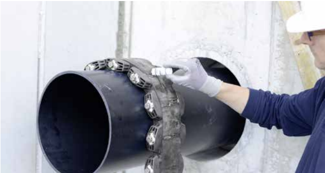
GKD400 - installation preparation with lubricant GM
