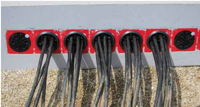
low-voltage cables sealed with HSI150 DG 6x10-36
