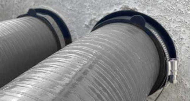
HSI150 KMA, single sealing packing with hinged rubber sleeve, Hateflex connection
