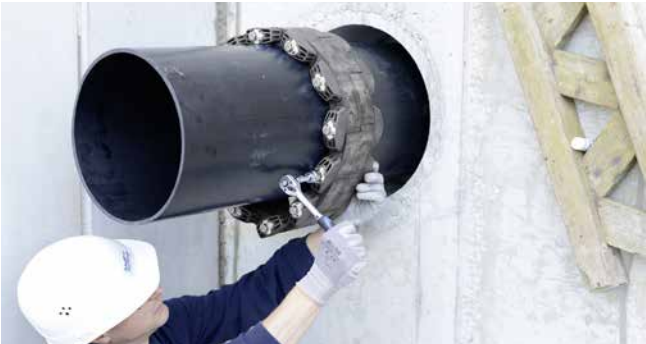
GKD400 - tightening of segments
