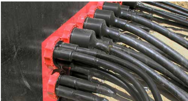
station entry: low-voltage cable sealed HSI90 D1x75 WS and HSI90 D3x32 WS
