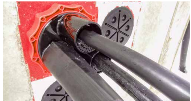
centring tape in system cover plugs of HSI150 D3x58 WS
