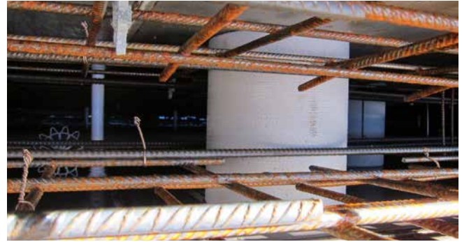
ZVR200/300 fixed in formwork
