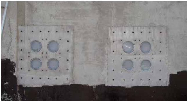
concreted fixed flange of the double wall insert HSI150 2x2 FLFE/X
