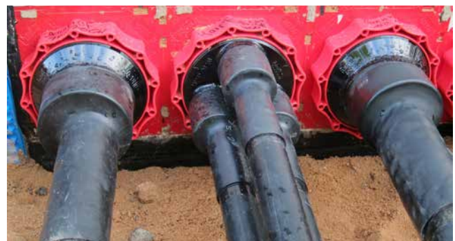
centring tape in system cover plugs of HSI150 D3x58 WS
