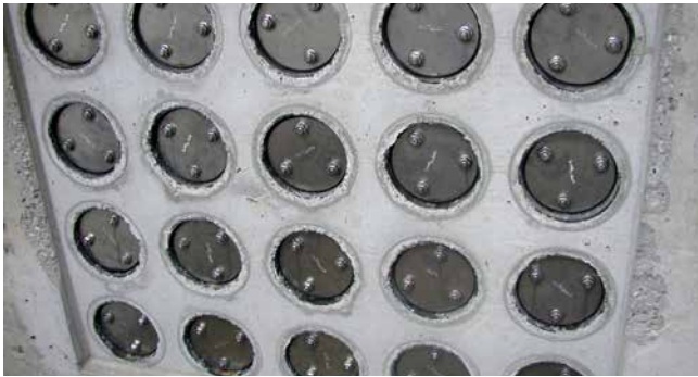
FZR100/240 - pipe section sealing
