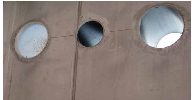
ZVR200/300 fixed in formwork
