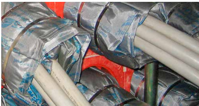
HSS - installation fire-stop pads in wall insert HSI150-K2, sealing with system cover or SEG-MENTO
