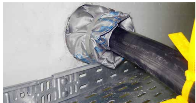
HSS - installation in core drill hole with HRD press seals
