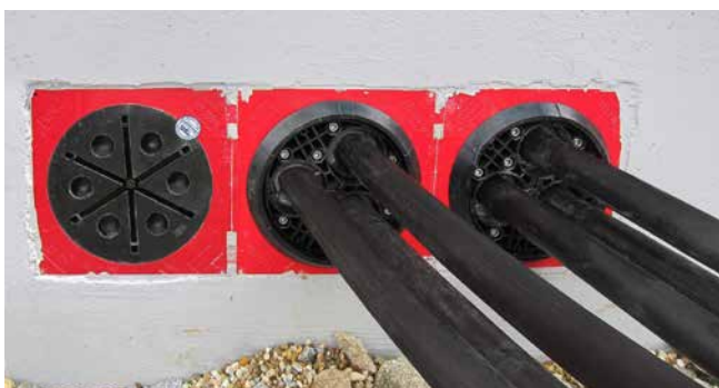
various installation stages for HSI150 DG 3x24-54
