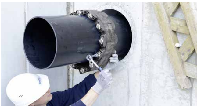
GKD400 - tightening of segments
