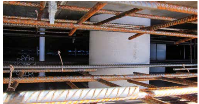
ZVR200/300 fixed in formwork
