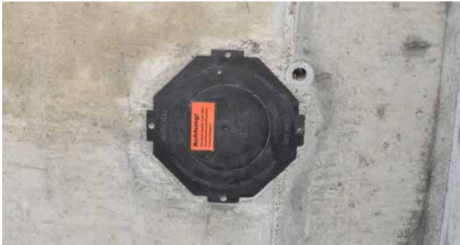
Practical picture of UDM/UDME in concreted wall
