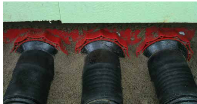
connection of corrugated pipes with cold shrink sleeves HSI150 D1x110 KS WR
