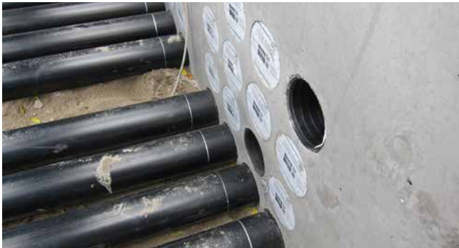
HSI150 GSM Varia applied as a block
