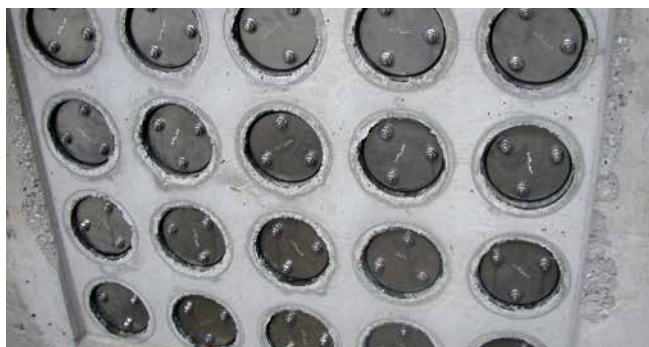
FZR100/240 - pipe section sealing
