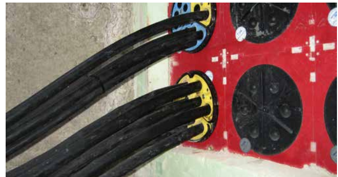
sealing of cables for street lighting with SEGMENTO
