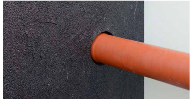
Practical image of UDM/UDME installed with PMBC coating and connected KG pipe
