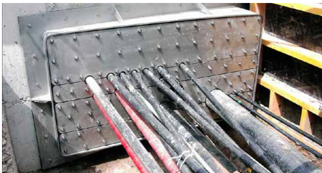
rectangular split flange for several cable penetrations
