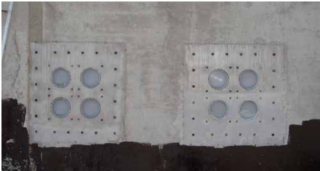
concreted fixed flange of the double wall insert HSI150 2x2 FLFE/X
