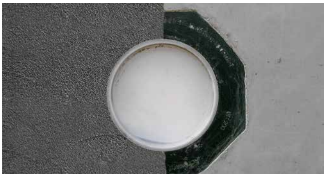
concreted UFR with PMBC
