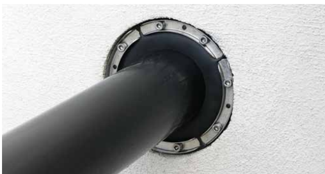
HSD200 1x159 b20 A2/EPDM55 "shaft seal"
