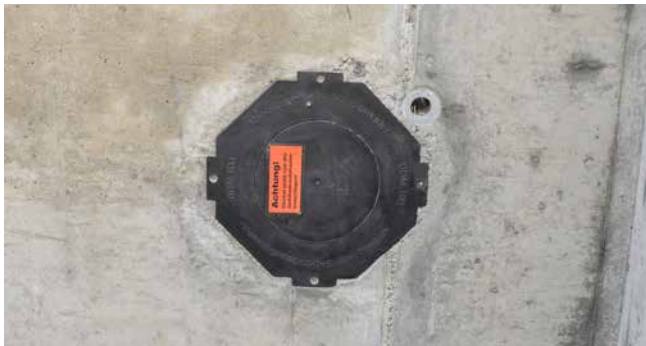
Practical picture of UDM/UDME in concreted wall
