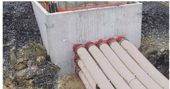
KES MA90 D - connection to the HSI90 wall insert
