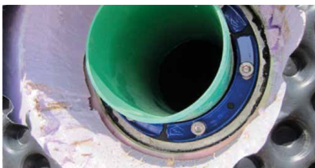
HSD150 C 1x110 b40 A2/EPDM55 in galvanised fixed/loose flange
