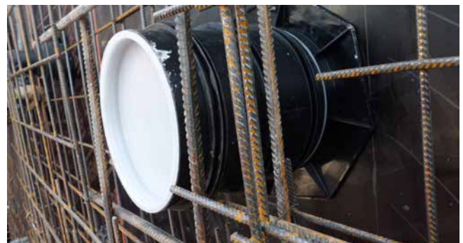
UFR in formwork
