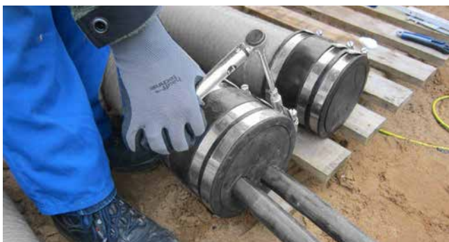
pressure-tight connection of spiral hose Hateflex14090 to wall insert HSI90 and end stop for the cable duct
