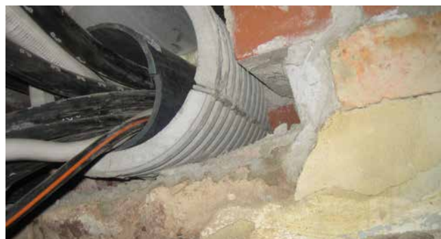
FZRG150/350 - refurbishment in masonry
