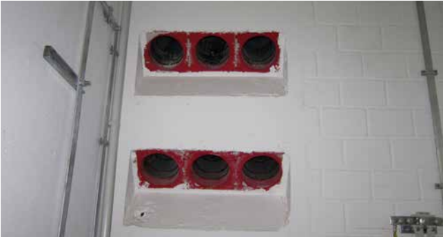
section 2x HSI150 1xZ K2 S45°/X double wall insert
