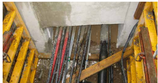
existing rectangular recess - has to be subsequently sealed
