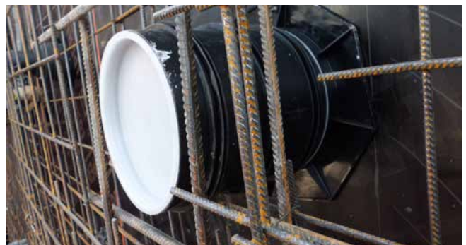
UFR in formwork
