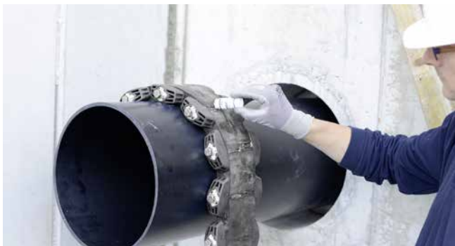
GKD400 - installation preparation with lubricant GM
