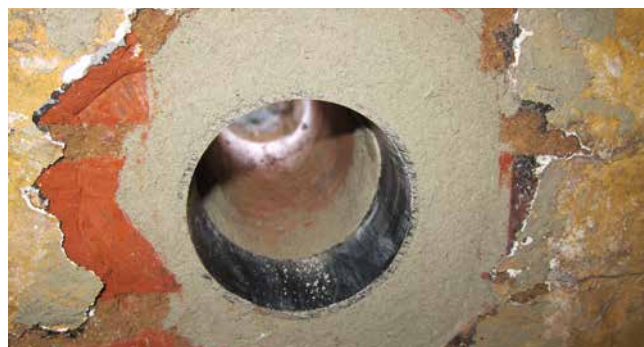
SFR subsequently incorporated into the masonry
