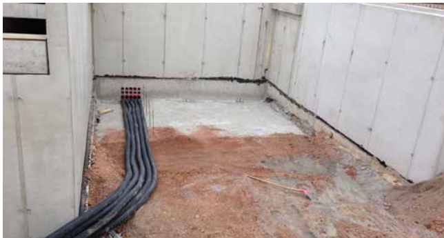
connection of corrugated ducts HSI90 D1x75 KS WR
