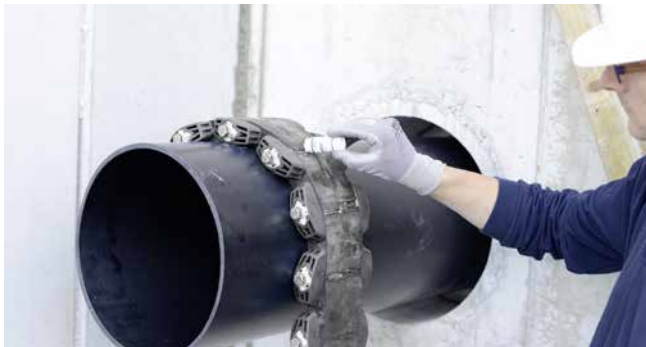
GKD400 - installation preparation with lubricant GM
