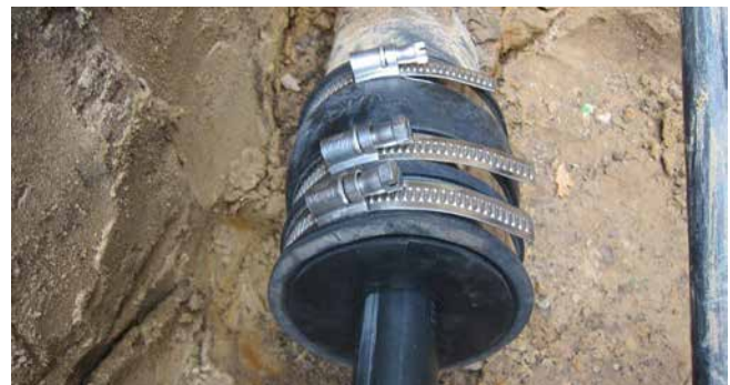
sealing set KES90 MA WE100 SG 1x18-65 SET for cable sealing at end of cable duct
