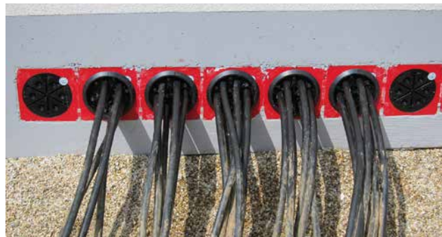
low-voltage cables sealed with HSI150 DG 6x10-36
