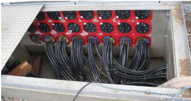
HSI150 - wall inserts fitted with SEGMENTO sealing for control cables in a transformer house
