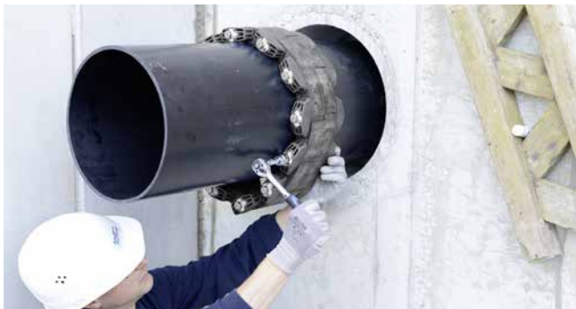
GKD400 - tightening of segments
