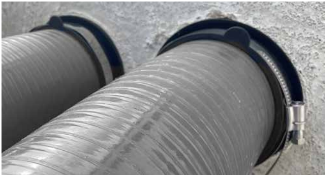
HSI150 KMA, single sealing packing with hinged rubber sleeve, Hateflex connection
