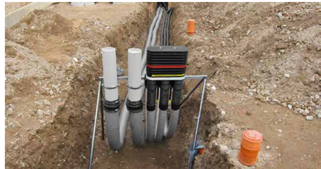
side by side arrangement 2x KES90 MA ZVR100/500 on the installation fixture KES FUBO-FIX AV
