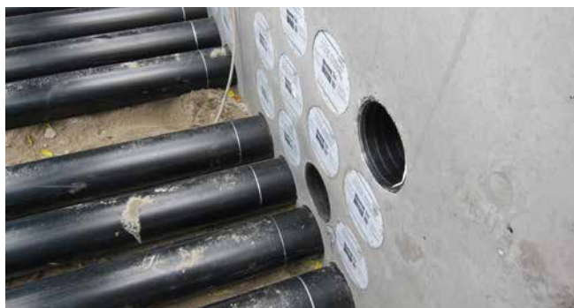
HSI150 GSM Varia applied as a block
