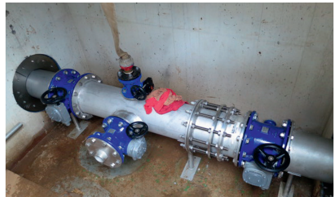
HRD seal and stainless steel flange T-fitting with shut-off valve and venting valve
