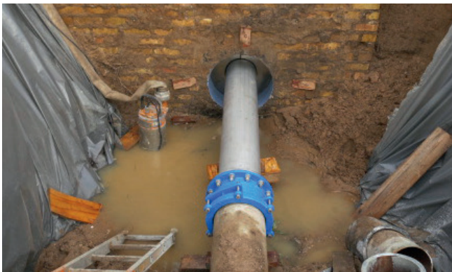
HRD seal installed in the core drilled hole with centered stainless steel pipe
