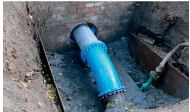
construction pit with prepared underground and concreted support foundation to avoid settlement.
