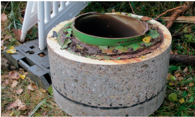
core of the 800 mm core drill with the old steel pipe
