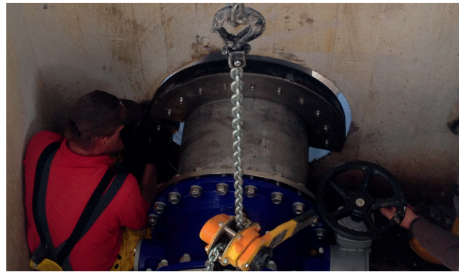
installation of the split press seal HRD for sealing the stainless steel pipe in the core drilled hole
