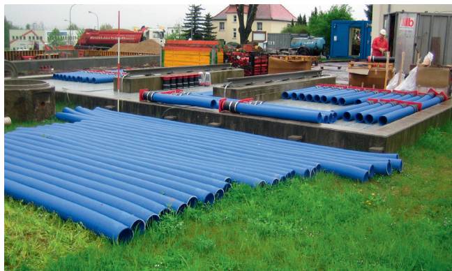
Coordination of material – Installation of Hateflex spiral hose 14150 with sleeve system. The system is laid out at the ramp to ease the allocation to the concrete basement.
