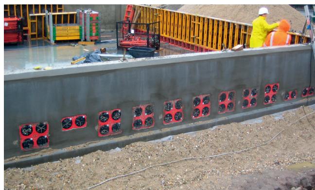
Laying of system – Connection to the already cast-in double wall insert HSI 150-K2/250 to achieve the sealing on both sides.
