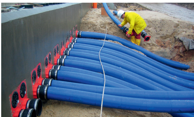
Laying of system – Connection to the already cast-in double wall insert HSI 150-K2/250 to achieve the sealing on both sides.
