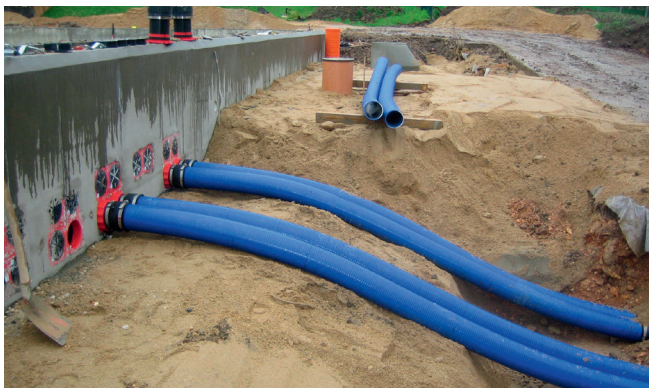
Laying of system – Connection to the already cast-in double wall insert HSI 150-K2/250 to achieve the sealing on both sides.
