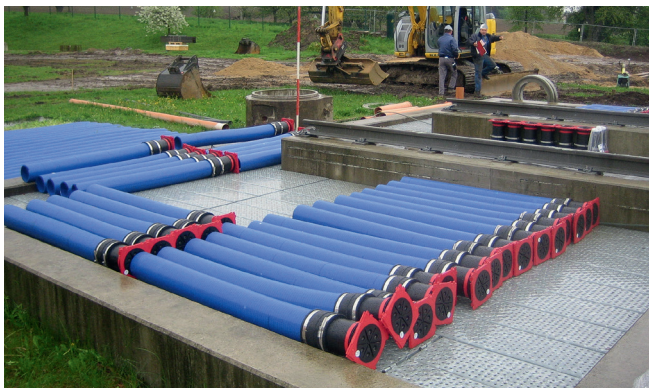
Coordination of material – Installation of Hateflex spiral hose 14150 with sleeve system. The system is laid out at the ramp to ease the allocation to the concrete basement.
