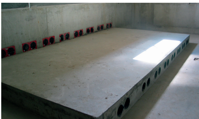
Connection to HSI 150 cable entry system – Connection of Hateflex spiral hose with sleeve system – for elongation and lowering of connections.
