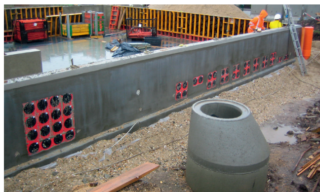
Connection to HSI 150 cable entry system – Connection of Hateflex spiral hose with sleeve system – for elongation and lowering of connections.
