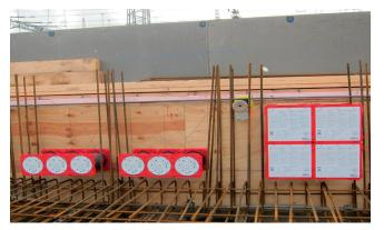
Wall inserts HSI 90 and HSI 150 and earthing entries are installed in theformwork.
