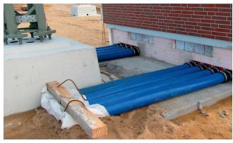
Wall inserts HSI 150 are set in concrete and KES-systems 14150 are connected to the wall inserts using sleeve method.
