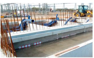
Flexible cable duct systems KES-M 150 using Hateflex 14150 and KES-M 90 using Hateflex 14090 are being laid.
