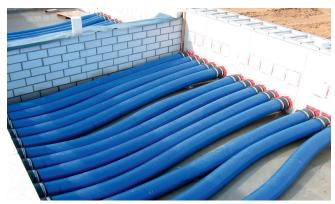
Wall inserts HSI 90 are set in concrete and KES-systems 14090 are connected to the wall inserts using sleeve method.
