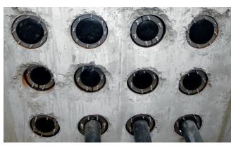
Using universal press seal elements, standard openings provided by individual cable arrangements are easily, quickly and securely sealed.
