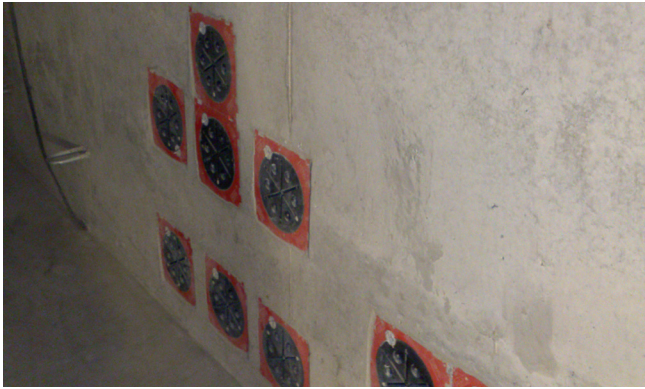
Hauff-Technik wall inserts after concreting in completely dry cable trench.
