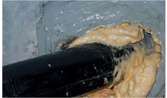
Old sealing methods: Use of 2 types of organic sealants due to the failure of the first attempt failed.
