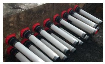
Connection of rigid Telstra conduits to HSI 150 wall inserts using KES-M 150-D system cover
