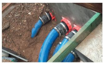
Connection of Hateflex spiral hose using KES-M 150-D system cover
