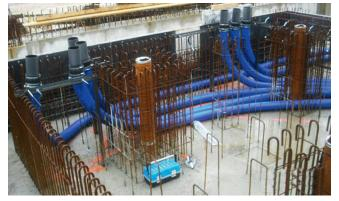
Cable entry system KES-M 150 as water pressure tight and flexible lead through the bottom slab.
