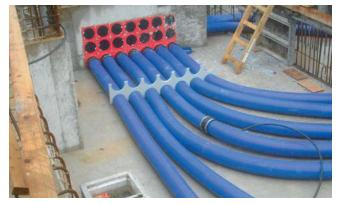
Cable entry system KES-M 150 with spacer for fixation and positioning of the hose bundels.
