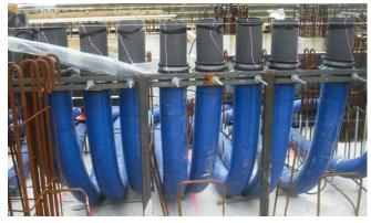
Precise alignment of the KES-M 150 system and the pipe sockets at the top of the finished floor level. Precise alignment with the top level of the flooring can be achieved by cutting to length the pipe sockets.
