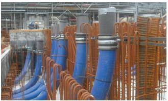
Cable entry system KES-M 150 with renovation wall sleeve SFR. Lead through the planned bottom slab for a pressure tight empty duct connection to the cable pits and for continuative laying in the ground of power and control cables.
