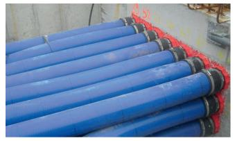
Cable entry system KES-M 150 with pressure tight connection to the concreted wall insert HSI 150-K2.
